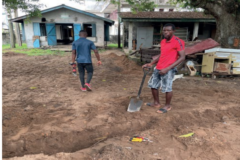
digging for grounding
