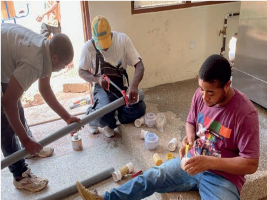
Aminu connects the sewage pipe
